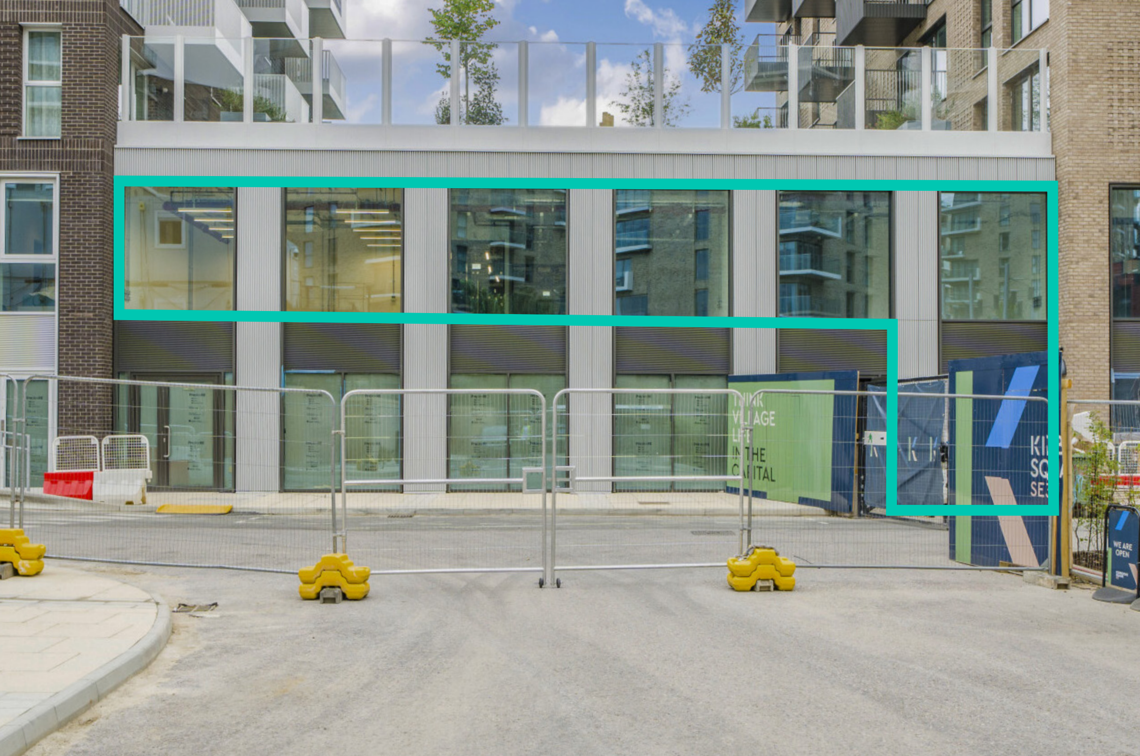
Photo of first floor office accommodation with retail below
