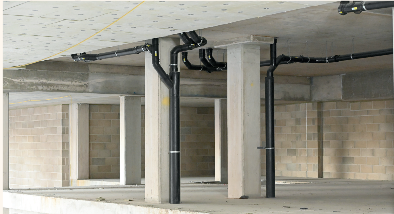
UNIT 3.B20 MEZZANINE
